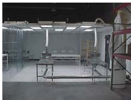
Overview picture of two stations including air knives and vacuum collection located under each air knife.
