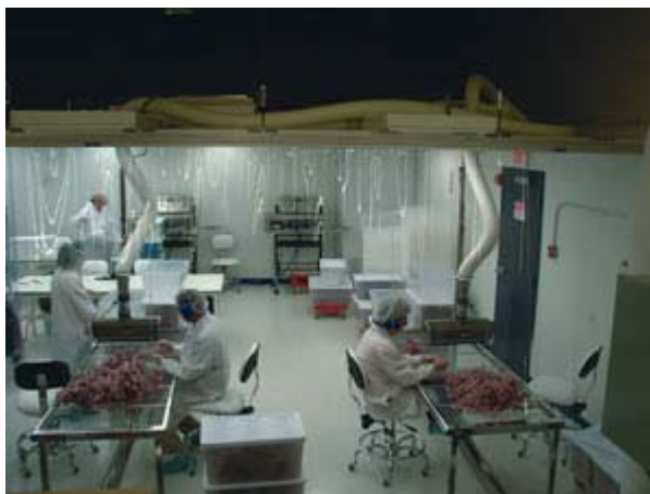
Overview of a cleanroom with ionizing air knives
